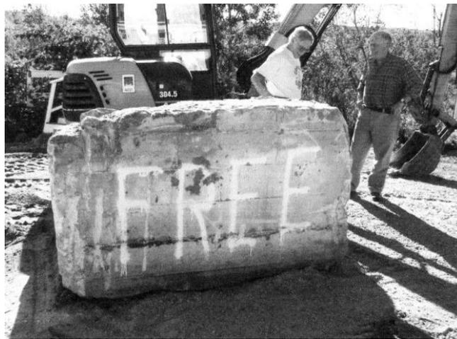
Believe it or not, there was a taker for this ten-ton block of concrete, which had been a part of the original steps to our museum. It had to be removed because it was exerting pressure on the basement wall, causing it to bow and crack. Phil Barker and Bob Evans pondering on how to get rid of it.
